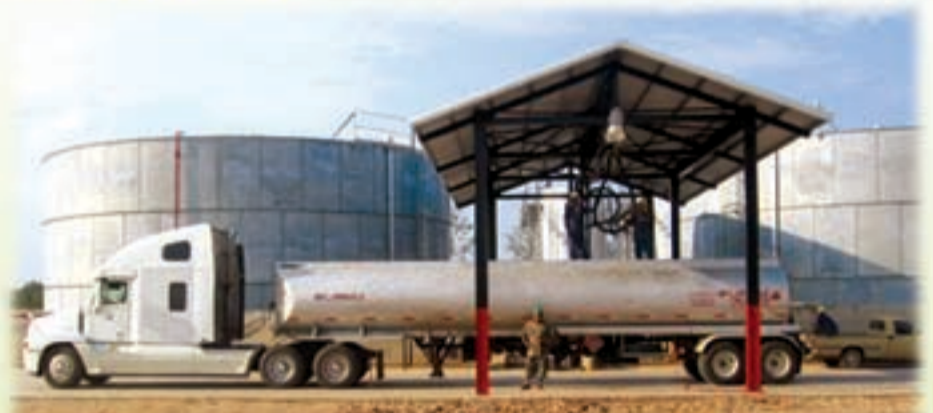
Oil storage and truck loading bay at Iguana Creek
