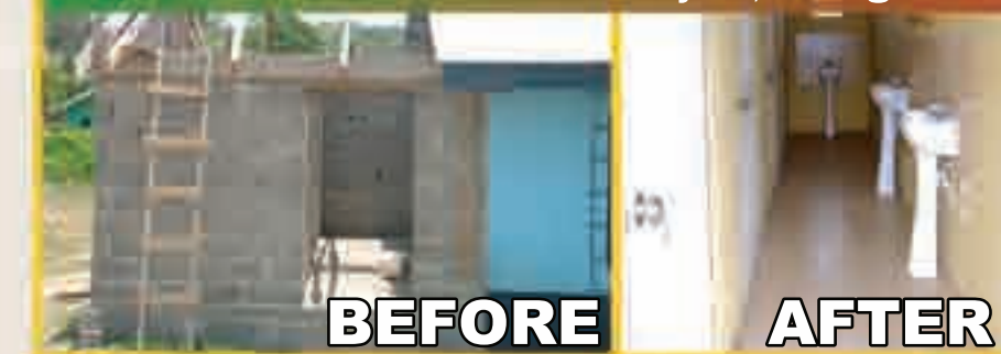
St. Hilda's School Bathroom Project, Georgeville
