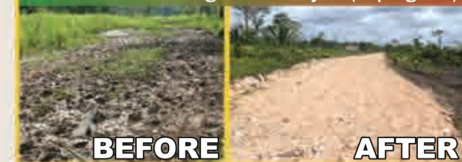
More Tomorrow Village Road Project (in progress)
